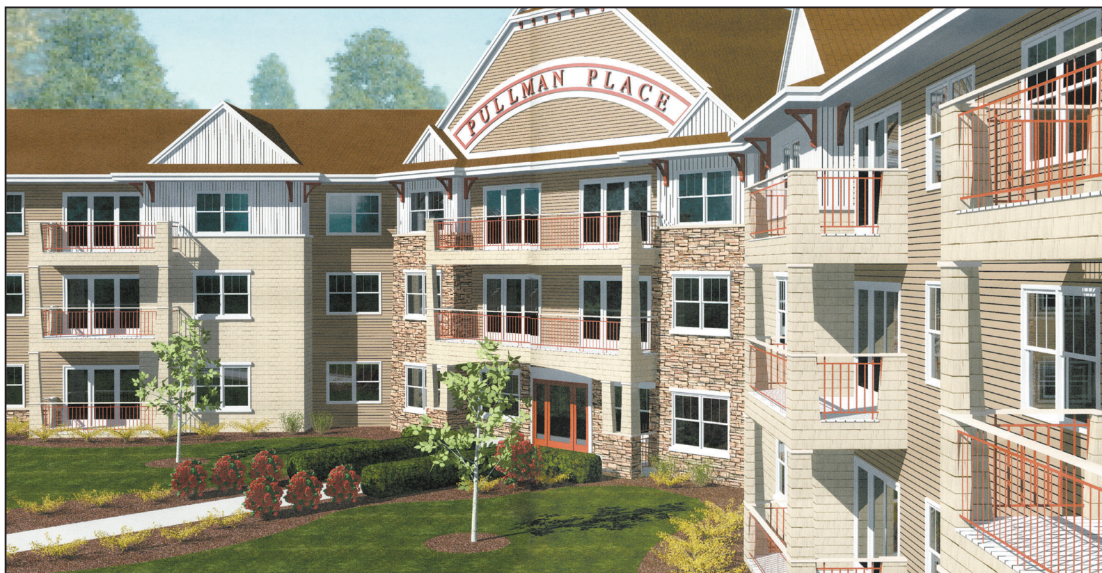
An artist's rendering of what Pullman Place will look like. The senior housing cooperative will be built in Elk River.
